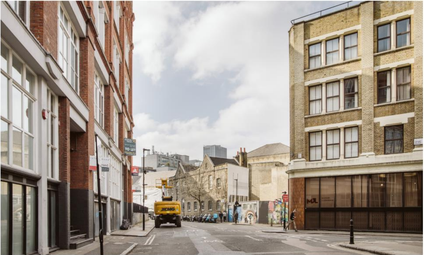
Image 3– View looking south along Tabernacle Street (former sixth form centre seen in centre to be demolished)
