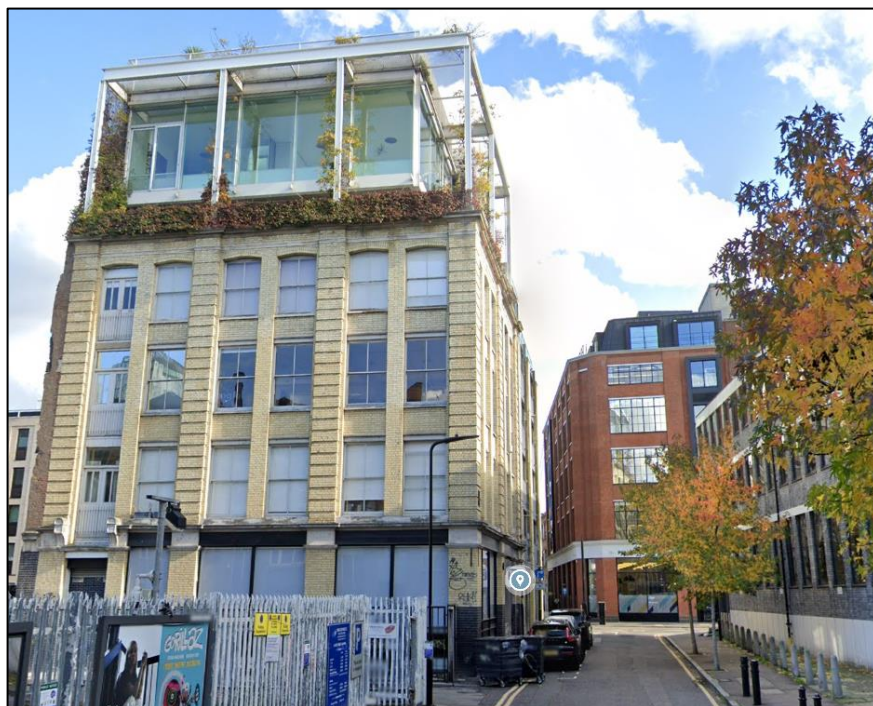
Figure 31: 17-18 Clere Street (western elevation)
