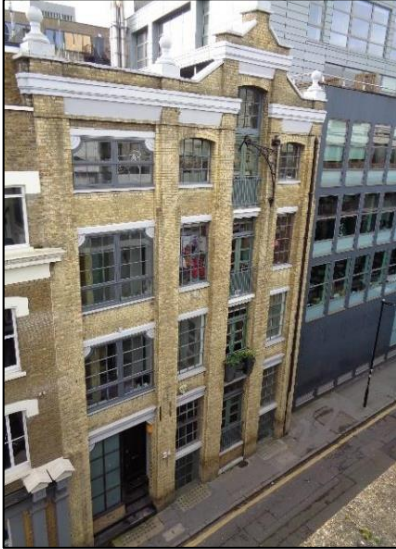
Figure 30: 17-18 Clere Street (western elevation)
