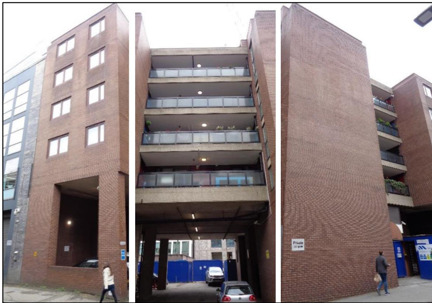
Figure 29: The principal elevation of 10 Epworth Street
